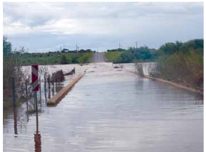
The low water bridge in Warrenton on Tuesday morning, 25/01/2011.
